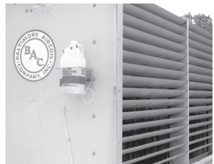
Arrange Drip Feeder so that weighted end is proper distance above or below surface of sump water.
